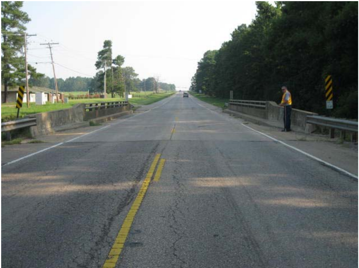
Note: No overlay on bridge deck
